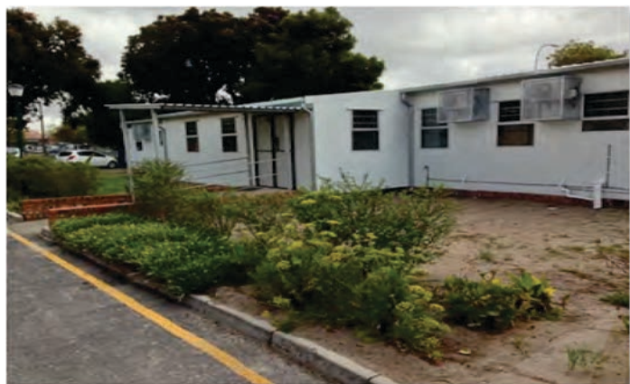
Example of a new TCC
